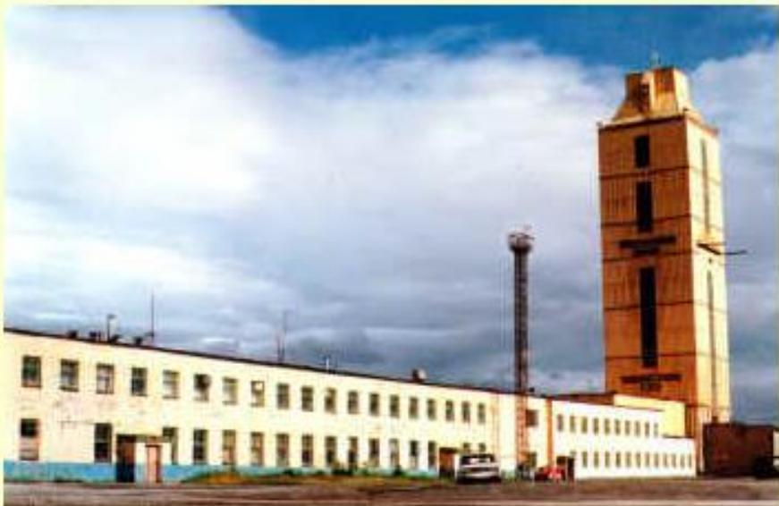
The 64-metre drill-rig enclosure over the 12-km-deep Kola borehole
