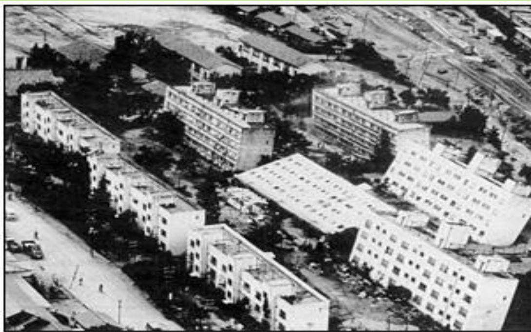
FIGURE 3 - THESE BUILDINGS IN JAPAN TOPPLED WHEN THE SOIL UNDERWENT LIQUEFACTION.
