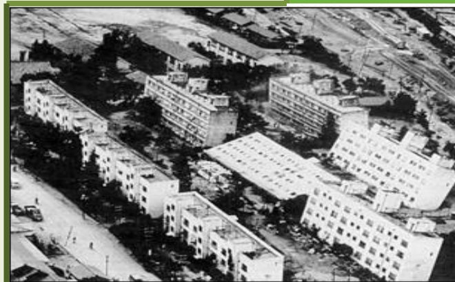
FIGURE 3 - THESE BUILDINGS IN JAPAN TOPPLED WHEN THE SOIL UNDERWENT LIQUEFACTION.
