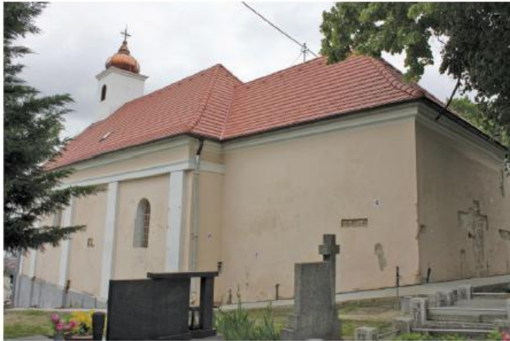
FIGURE 5 Photograph of church exterior (NW view from the cemetery).
